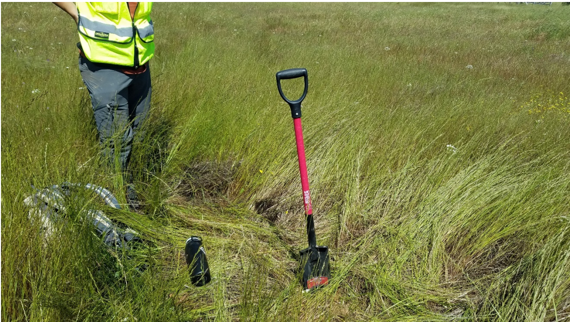
Arterial Roads Project. 170242
