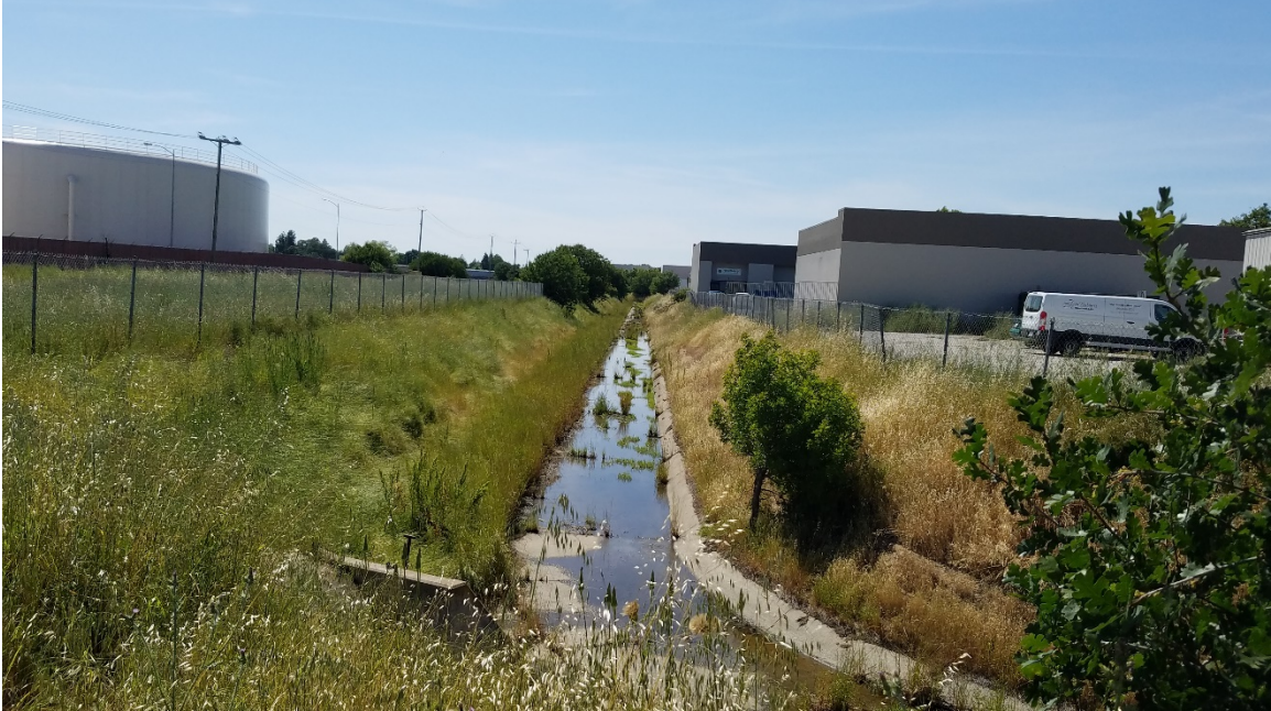
Arterial Roads Project. 170242
